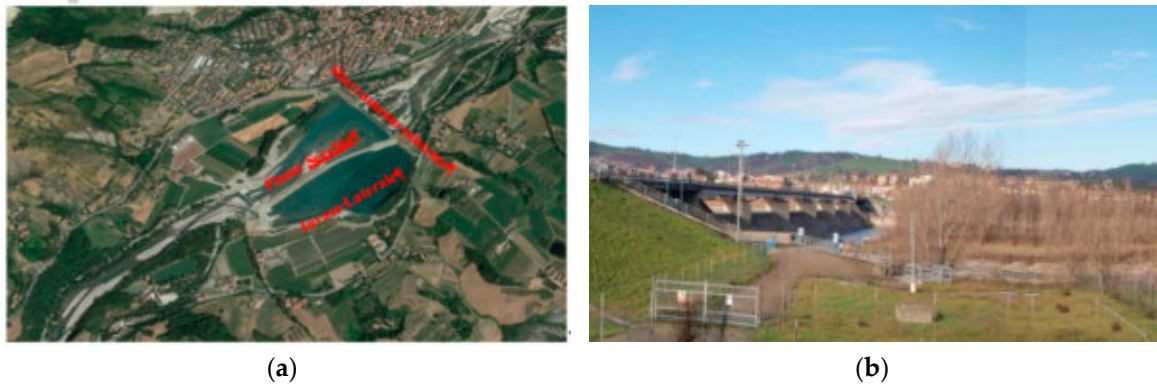
Figure 30. (a) photo of the current state-of-the-art; (b) photographic shooting of the downside of the weir.
