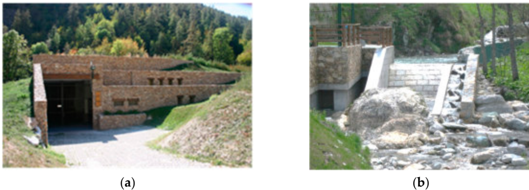
Figure 24. HPP “Frere 2” —Powerhouse (a) and intake works with the fish ladder (b).
