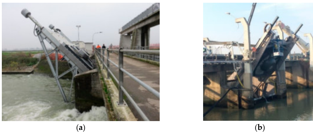
Figure 69. (a) Canda turbines during a flood; (b) Bussari turbine during maintenance activities.
