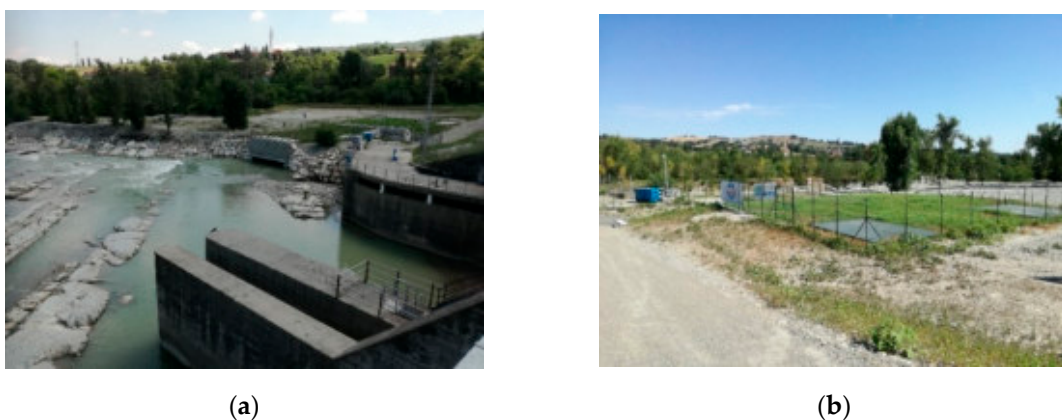
Figure 32. (a) photo from the upper side of the weir; (b) photographic shooting of the access to the building.
